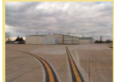
Leased Hangars (No. 10-13)
