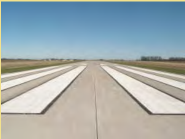
Runway 36 Threshold (Looking N)
